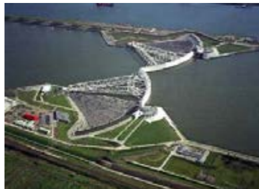
Maeslant storm surge barrier in the Nieuwe Waterweg (New Waterway)
