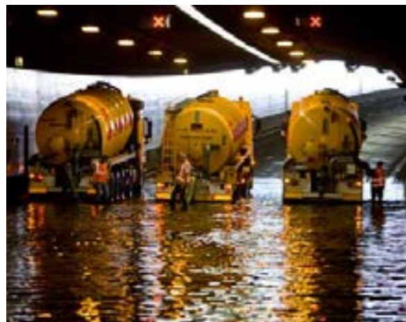
Flooding in the Botlek Tunnel in 2008 caused long traffic jams
