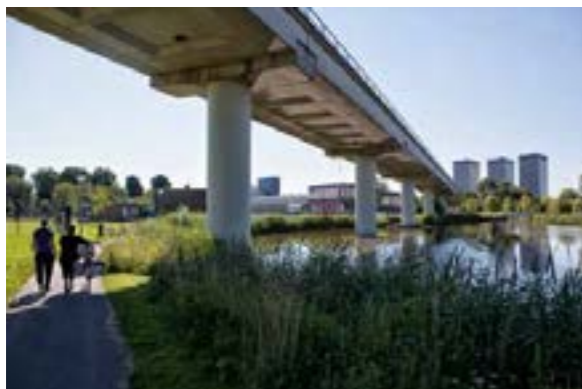
Extra surface water along the Tjalklaan
