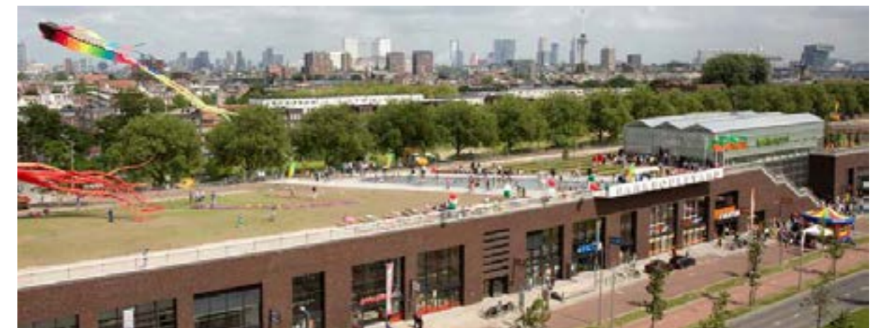
The roof top park Vierhavenstrip is a public outdoor area in a unique, multi-functional dike setting
