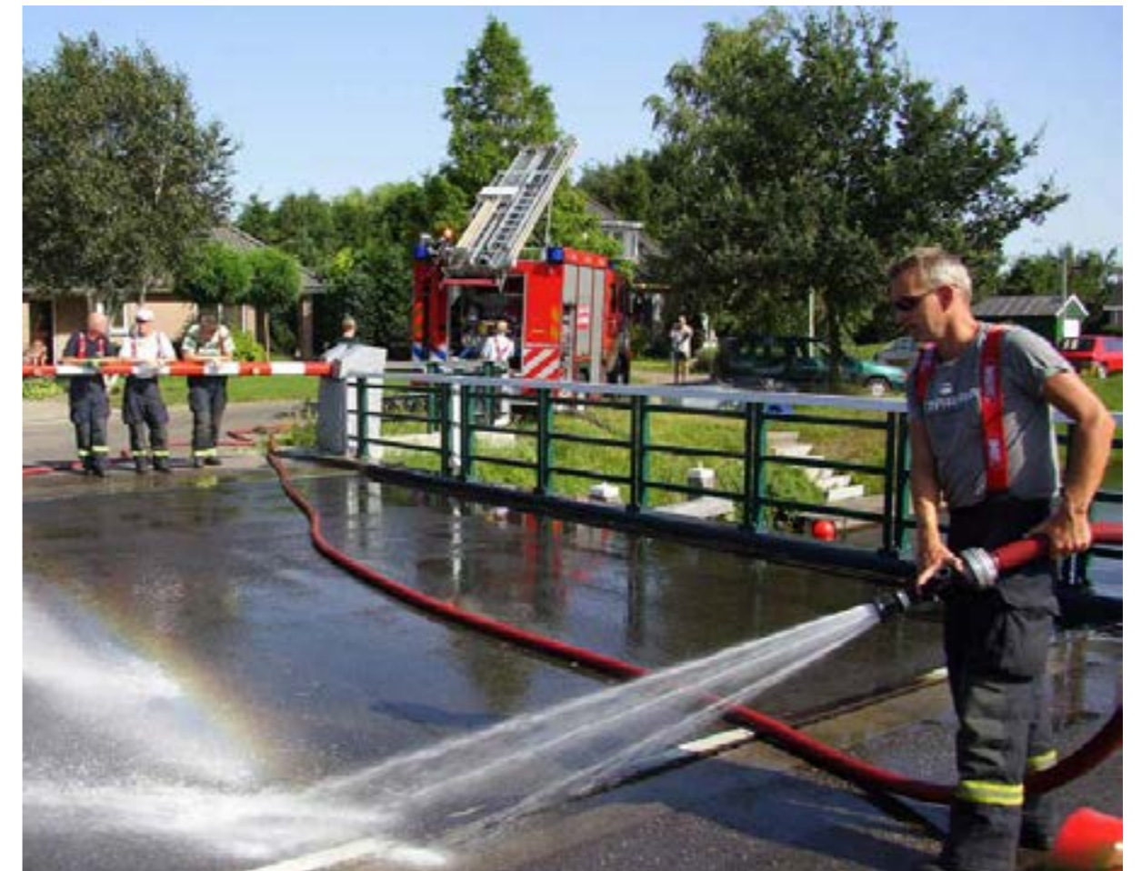
Spraying a bridge with water to prevent malfunctioning due to heat expansion
