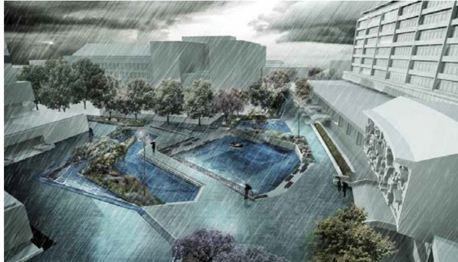
The Bentemplein water square as temporary water storage facility, artist's impression of the scene during a downpour
