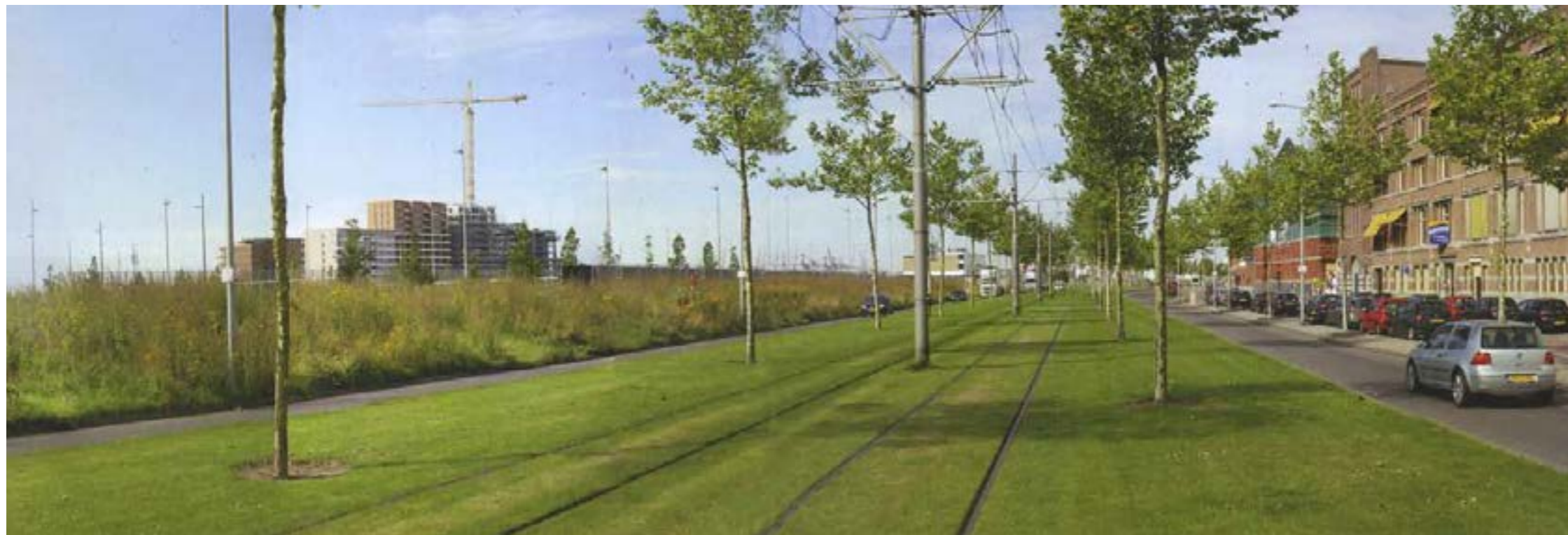
The primary dikes form an attractive green landscape with elevated cycle path along the Westzeedijk
