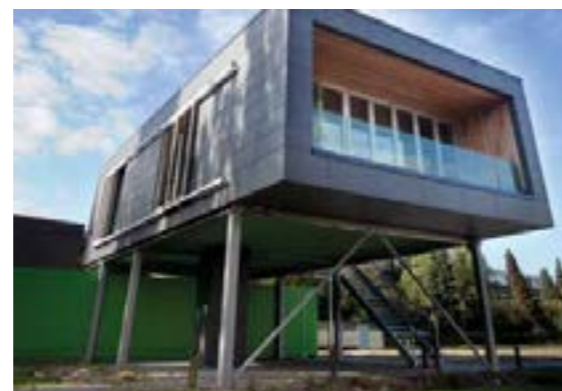
Concept House Village Heijplaat, flood-proof construction
